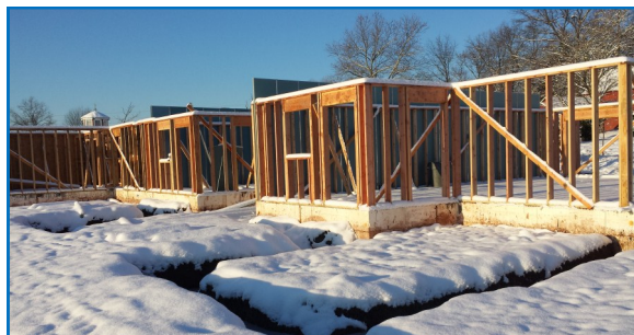
Penn Villa construction continues through a snowy winter.
